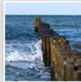
A groin is a short wall built at a 90-degree angle to the shoreline in an effort to collect moving sand. Normally, a beach will have several groins, or jetties, to trap sand moving parallel to the shoreline. Beach groins can be constructed from wood pilings, large rocks, or cement.
